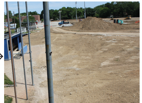
May 15, 2012 Construction begins on the new baseball field
