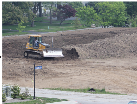
April 29, 2012 Bulldozers move dirt in preparation for the new stadium and softball field
